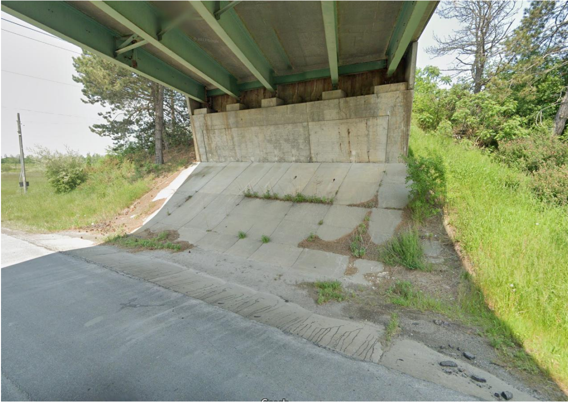
Photograph 3 – Abutment No. 2 (north side of existing bridge) supported on steel HP 12x53 piles.
