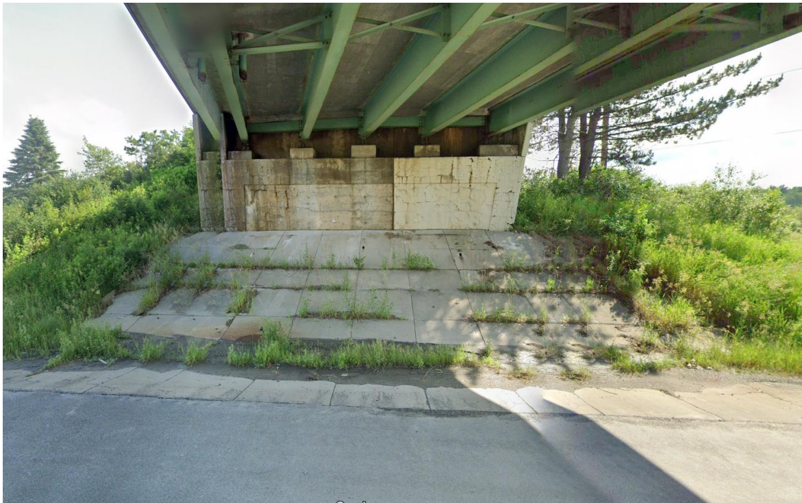
Photograph 1 – Abutment No. 1 (south side of existing bridge) supported on steel HP 12x53 piles.
